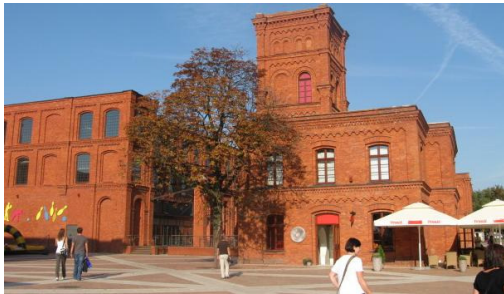
An example of the fine brickwork of the nineteenth century
